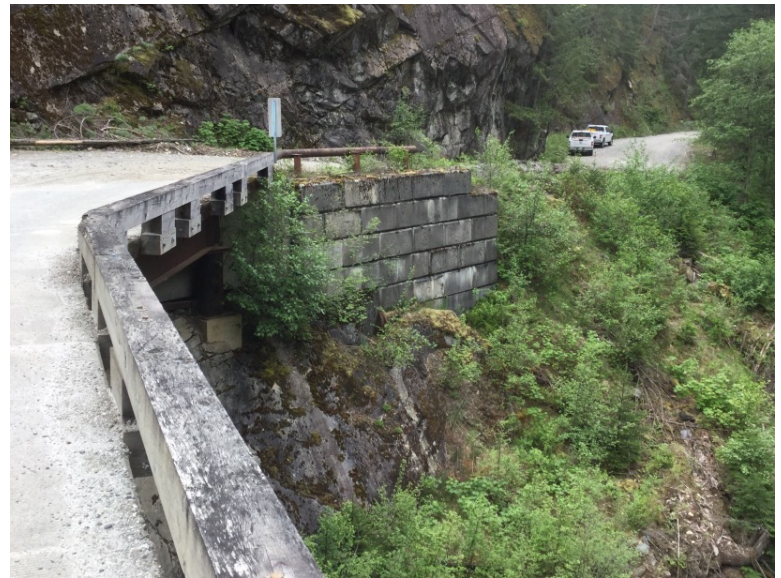
Downstream left bank retaining wall
