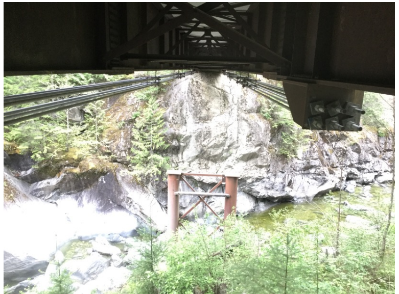
Right Bank Abutment when facing downstream
