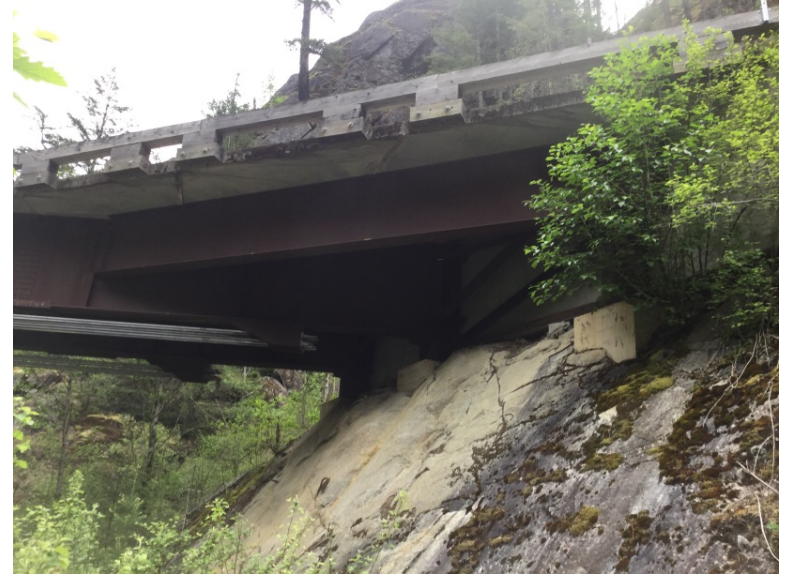
Left bank flared girder
